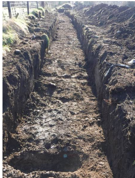
Plate 3 Trench 1 facing southeast
