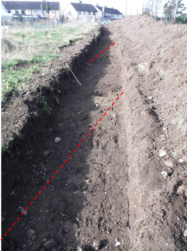
Plate 9 Trench 2, facing northwest showing the line of modern water pipe trench
